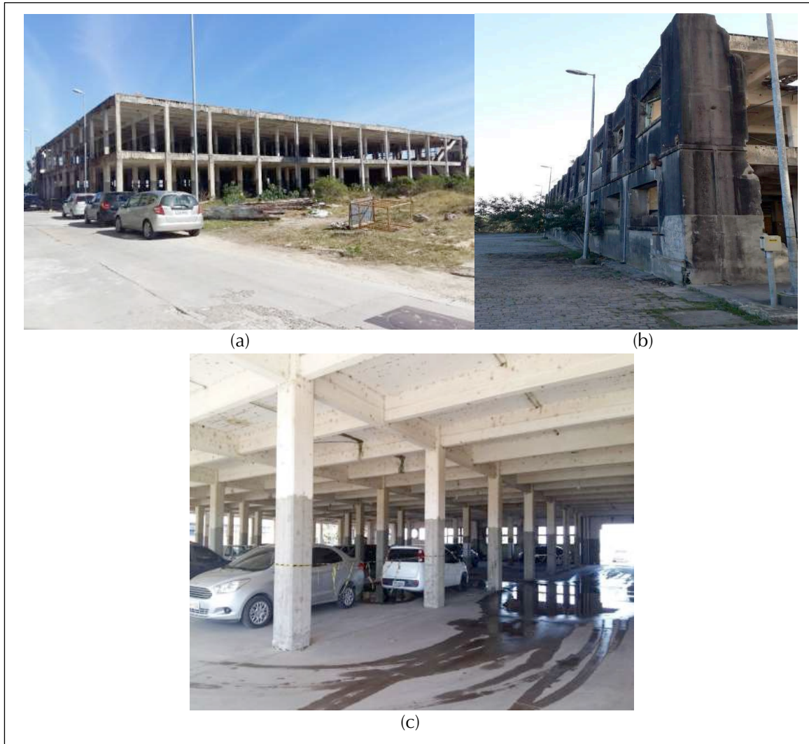
Figure 2. (a) North Facade. (b) South Facade. (c) Building used as parking
