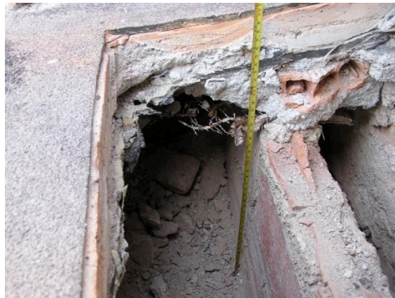
Figure 3. View of one of the test cuts on the rooftop of the building
