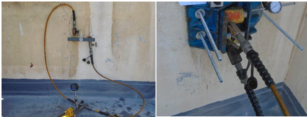
Figure 9. Tensile and shear testing of anchors
