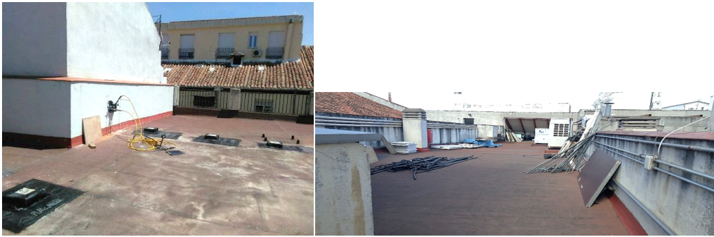
Figure 2. General views of the building rooftop
