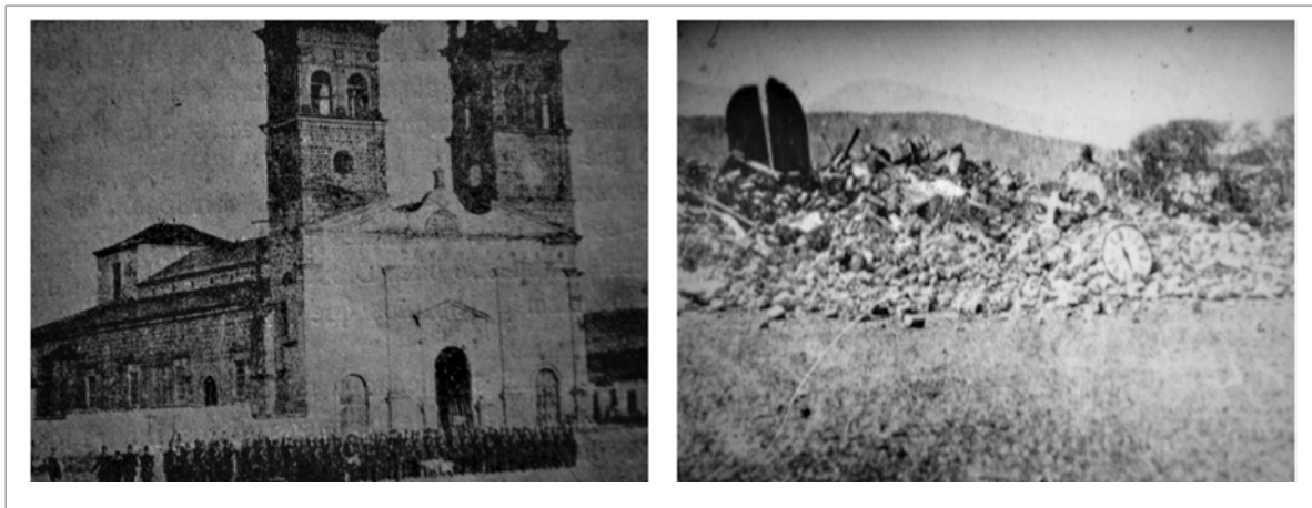
Figure 2. Collapse of the Cúcuta Church (made of earth) during the 1975 earthquake. Taken from (Ruiz et al., 2012)
