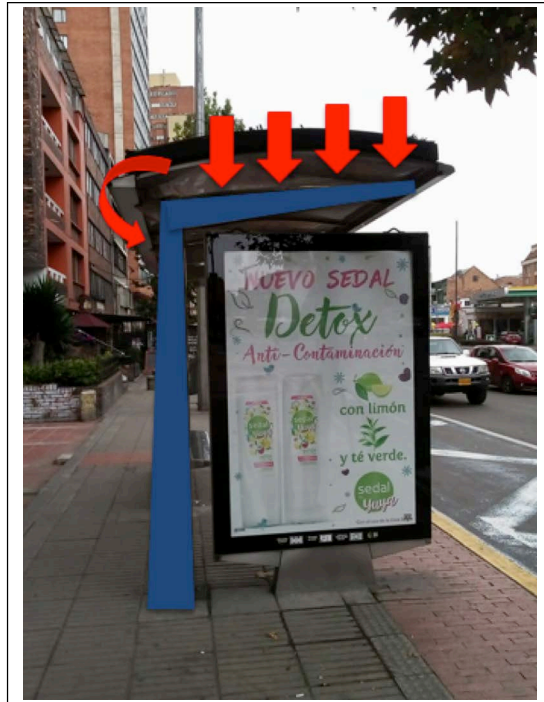
Figure 10. Representation of the green roof loading effect on the bus stop structure
