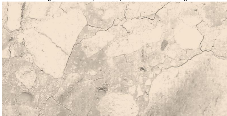
Figure 3. Cracks on specimen exposed 700 °C and air cooling.
