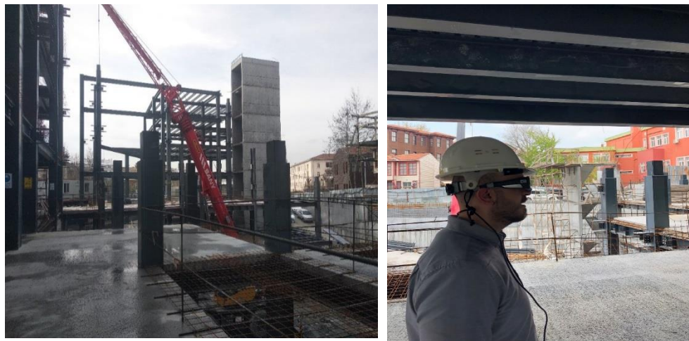
Figure 7. Construction site work area.
