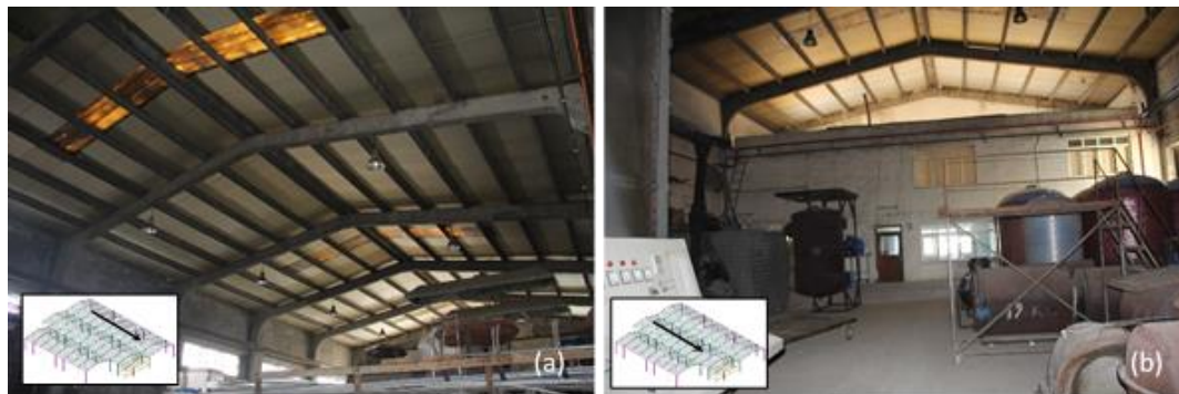
Figure 4. (a) inner view, (b) the view of administrative section.
