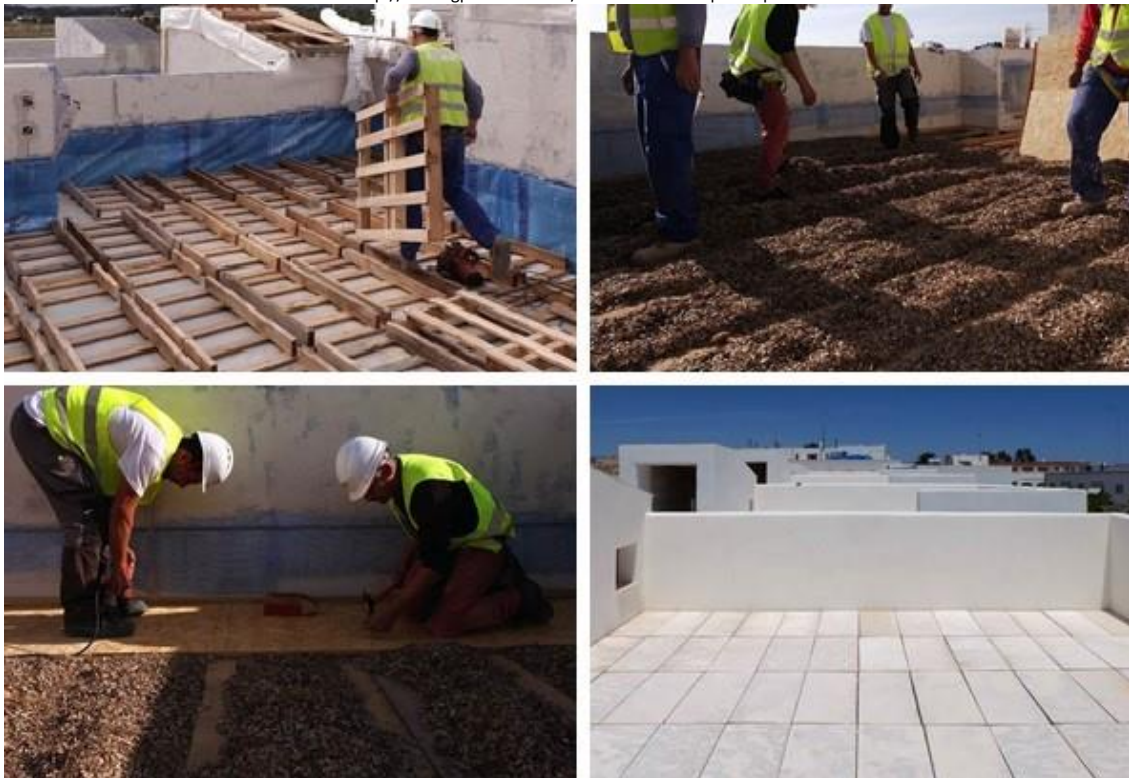
Figure 3. From right to left and top to bottom; positioning of the pallets on the waterproof sheet so they can be filled with the Posidonia; Filled with compacted Posidonia; Installation of the wooden boards (OSB/3) for containing the Posidonia; Final appearance of the finished rooftop; Source: taken from http://reusingposidonia.com/construccion-del-prototipo
