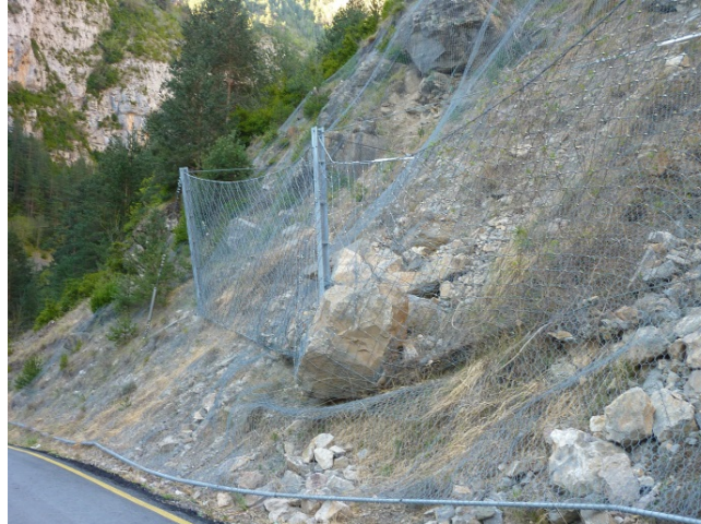
Figure 1. Example of dynamic barrier use for road protection. Source: R.L. Fonseca & Gonzalez-Gallego, 2007.
