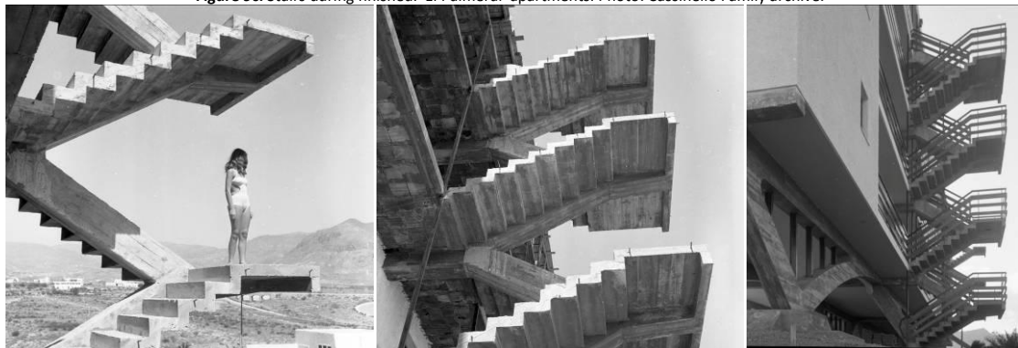
Figure 9c. Stairs during finished. 'El Palmeral' apartments. Photo: Cassinello Family archive.
