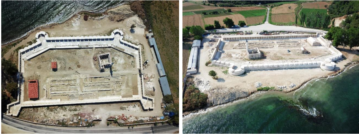
Figure 13. The aerial photo during rehabilitation process. Source: Authors.
