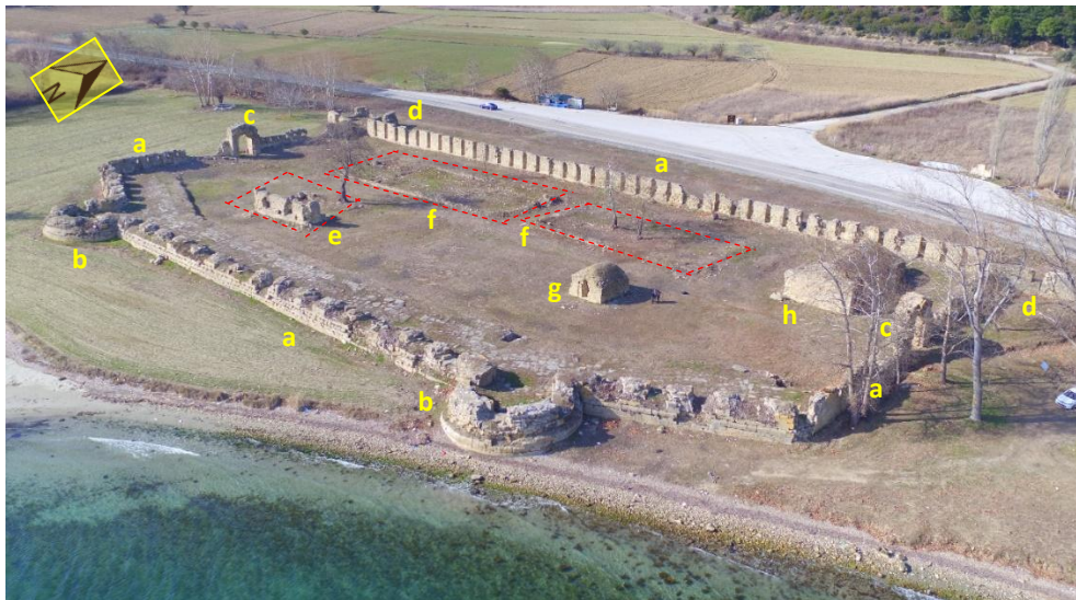
Figure 4. The current view of the ruined castle: a. Facades, b. Circular towers, c. West- and East-entrance, d. Square towers, e. Mosque, f. Military headquarters, g. Water fountain, h. Arsenal depot. Source: Authors.
