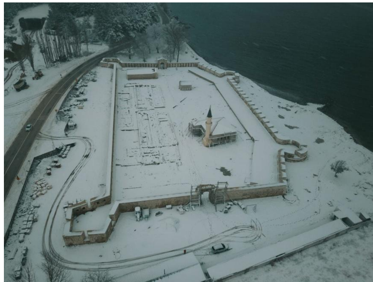
Figure 14. The overview after rehabilitation applications. Source: Authors.
